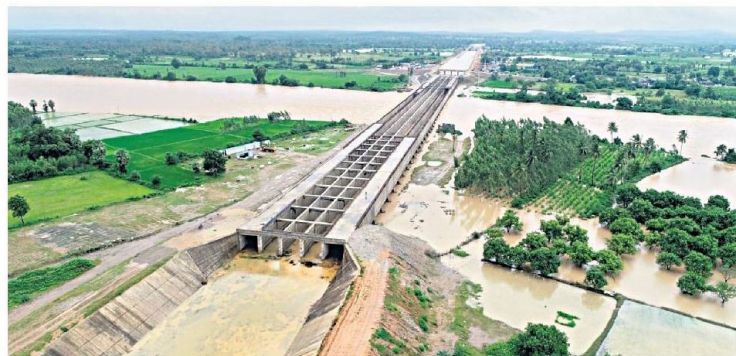
An aqueduct built across river Kinnerasani in Kothagudem district under package-3 of SRLI project.
