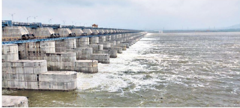
At Sundilla barrage, the inflows and outflows were 2 lakh cusecs as 60 of the 74 gates were lifted to discharge water downstream.
