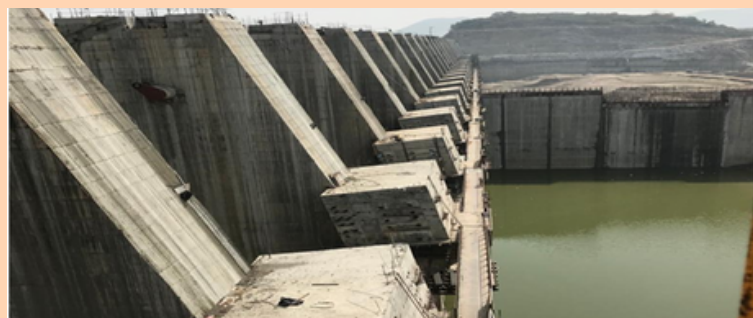
Prestressed trunion girder at Polavaram Irrigation Project, A.P
