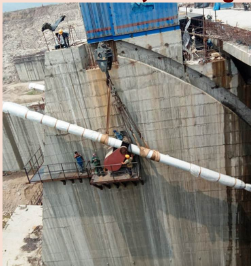
Erection of Hydraulic Cylinder
