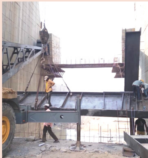
Erection of Bottom Horizontal Girder of Radial Gate
