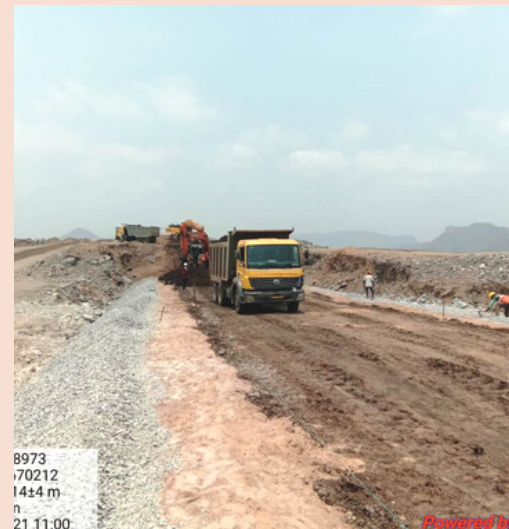
Upstream Cofferdam-Placement of Filters and Core
