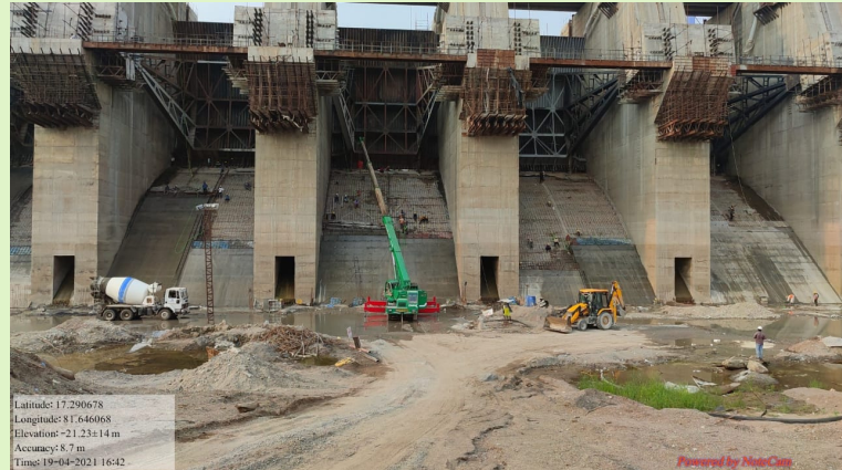
Polavaram Project, Andhra Pradesh - River Sluices- Concreting of Glacis
