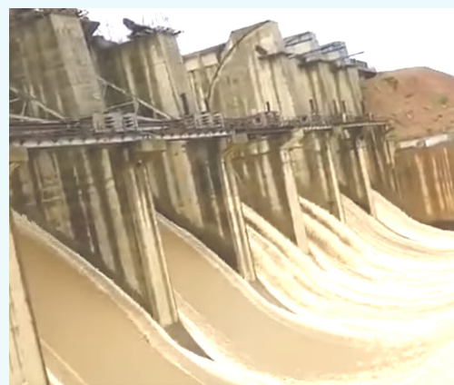
Halon Dam, 31m high, 1000 m long composite gravity dam in MP on Halon river, a tributary of the Narmada river. It provides irrigation facilities to about 13000 ha land. It was. The project was designed by CWC and commissioned last year.
