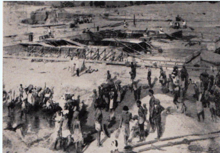
Gotta Barrage footage of piers 20 and 21 and excavation of foundation for pier 22 are seen here under construction.
