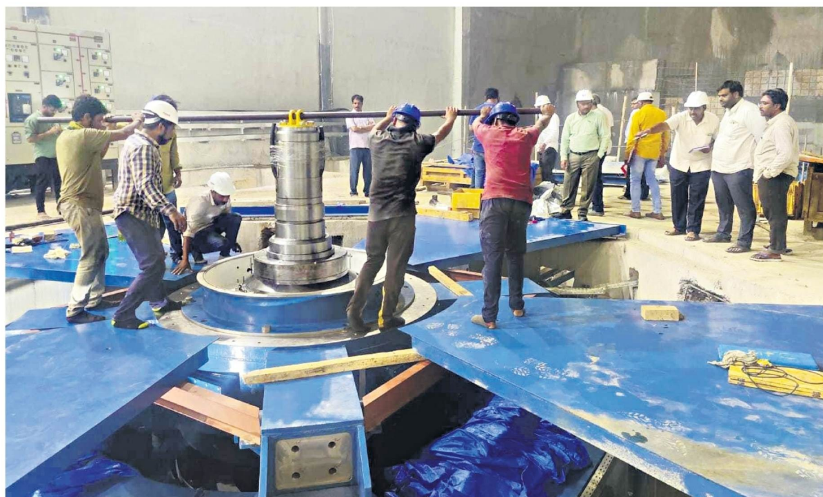
Workers fixing the motors at Malkapeta reservoir pump house. Godavari water to be pumped to the reservoir at Konaraopet mandal.
