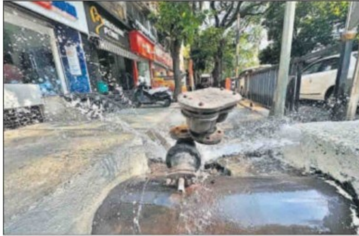
Thousands of litres of water being wasted due to leakage in the valve of a pipeline near TMC Office, in Thane. PRAFUL GANGURDE/HT PHOTO
