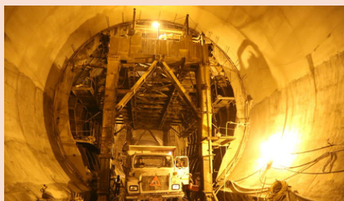
Completion of excavation of 6.3 km long HRT for Punatsangchu HEP-II in Bhutan having one of largest diameters (11m) in Asia
