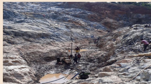
Shear zone in the foundation of the Non Over Flow portion
