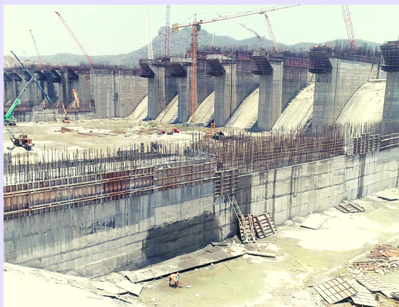
Ongoing Polavaram Project, Andhra Pradesh
