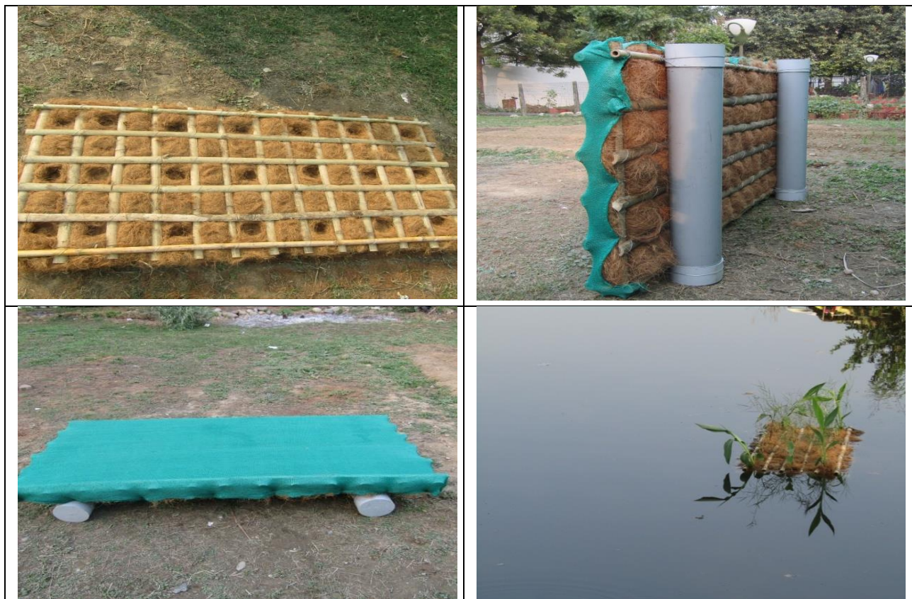
Figure 8.6: Construction of Floating Bed (Area: 50 m 2 ; 25 floating beds)
