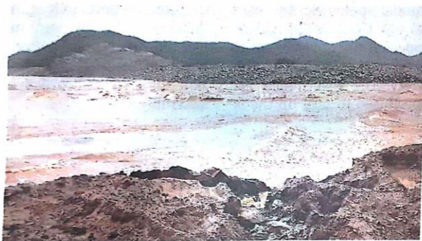
Safety concerns: Flood water at the Polavaram dam site flowing through the gap in the cofferdam. ■ A.V.G. PRASAD
