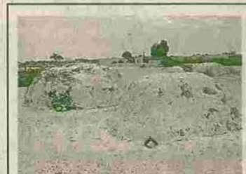
THE ORIGINAL FLYING SAUCER: The Kundi system in Rajasthan worked by paving the ground with lime, making it drain to the middle. When it rained, all the water got channeled into a well, kept covered to keep the water clean
