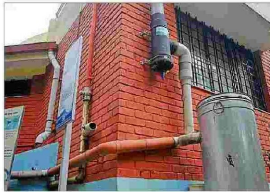
A rainwater harvesting system installed at a park in Jayanagar. DH FILE PHOTO
