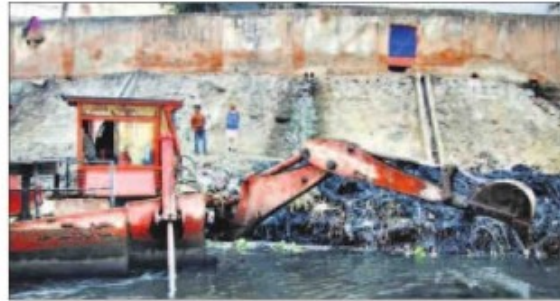
Desilting work underway at the Najafgarh drain. TWITTER/LTGGOVDELHI
