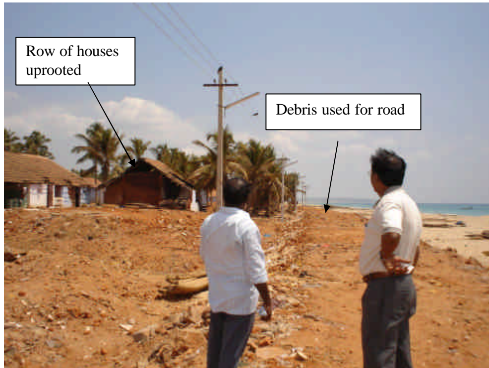
Photo 3.14 View showing a road formed with the debris removed along the coast at Kottilpadu
