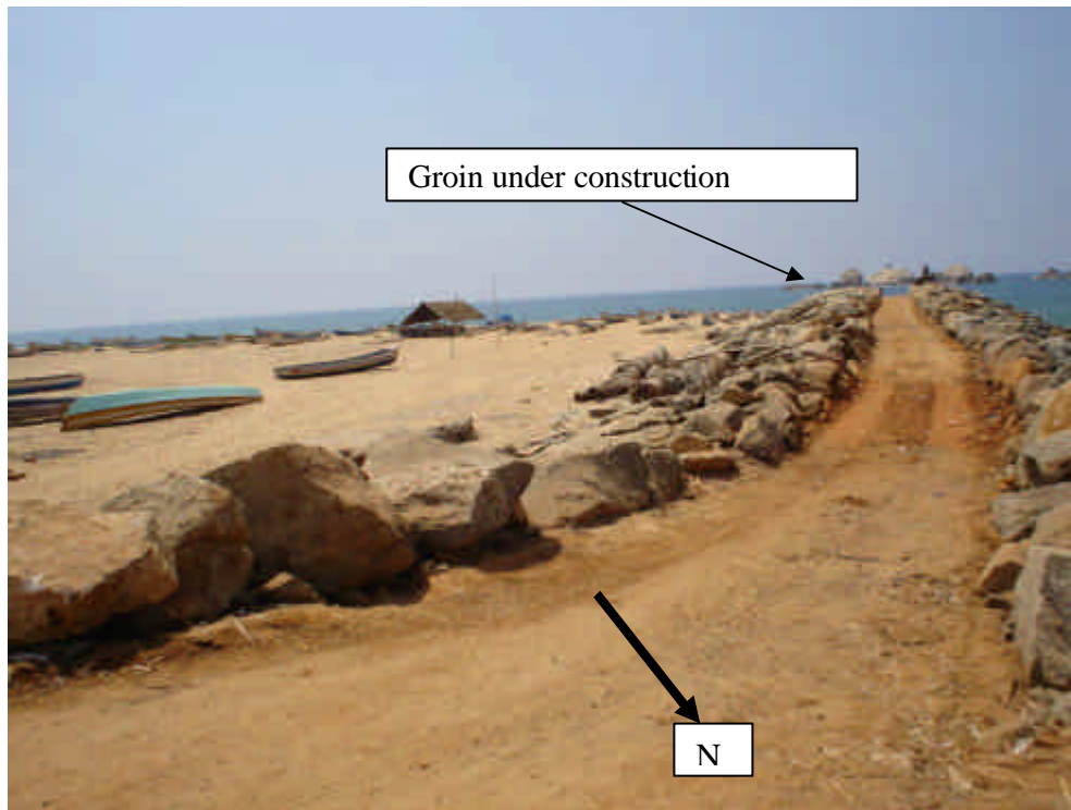
Photo 3.6 View showing the beach formed on the Eastern side of the groin under construction at Enayam
