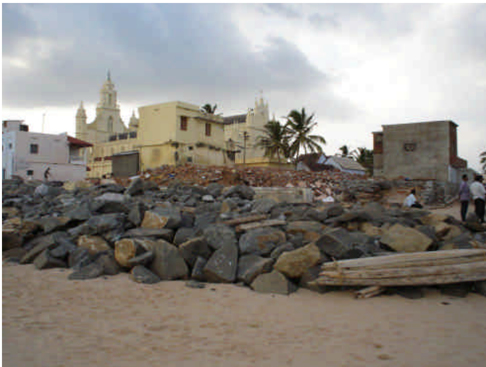
Photo 3.26. Erosion at the tip of the seawall
