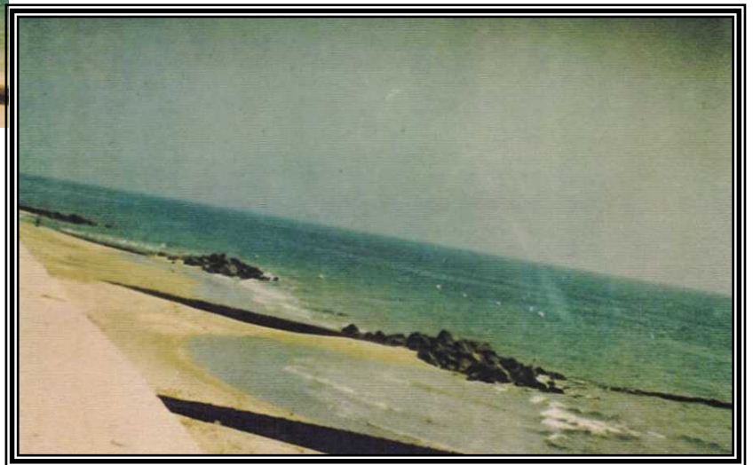
Photo. 1.8 T-Groin field protecting the coast of Florida
