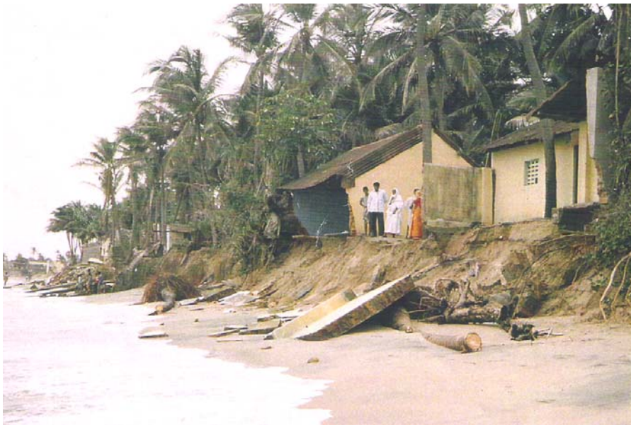
Photo 2.26. Damaged buildings due to coastal erosion at Rahamathnagar
