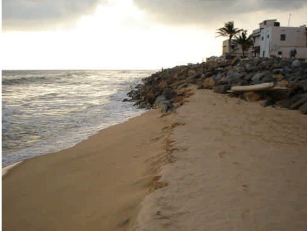
Photo 3.26. Erosion at the tip of the seawall
