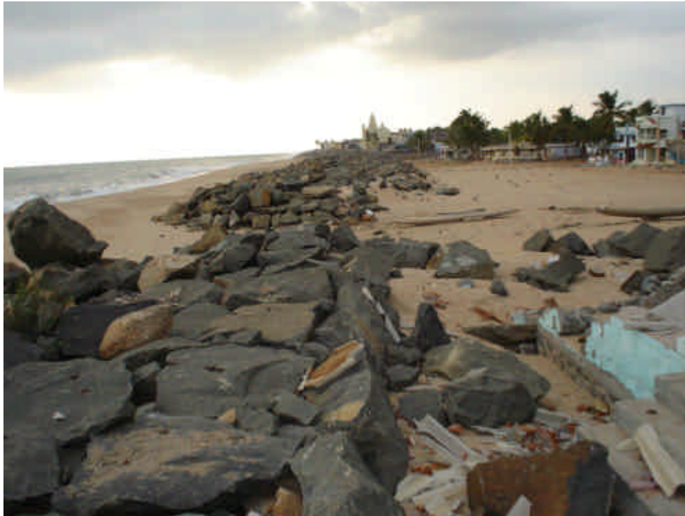
Photo 3.28. The damaged existing seawall at Keezhamanakudithurai
