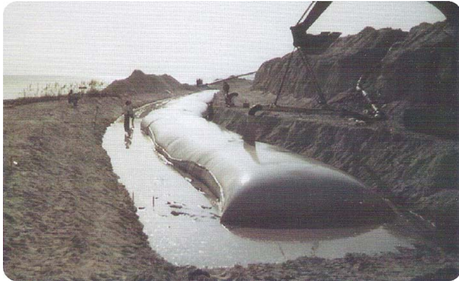
Photo. 1.5 Use of Geo-tubes to protect Island of Sylt, Germany
