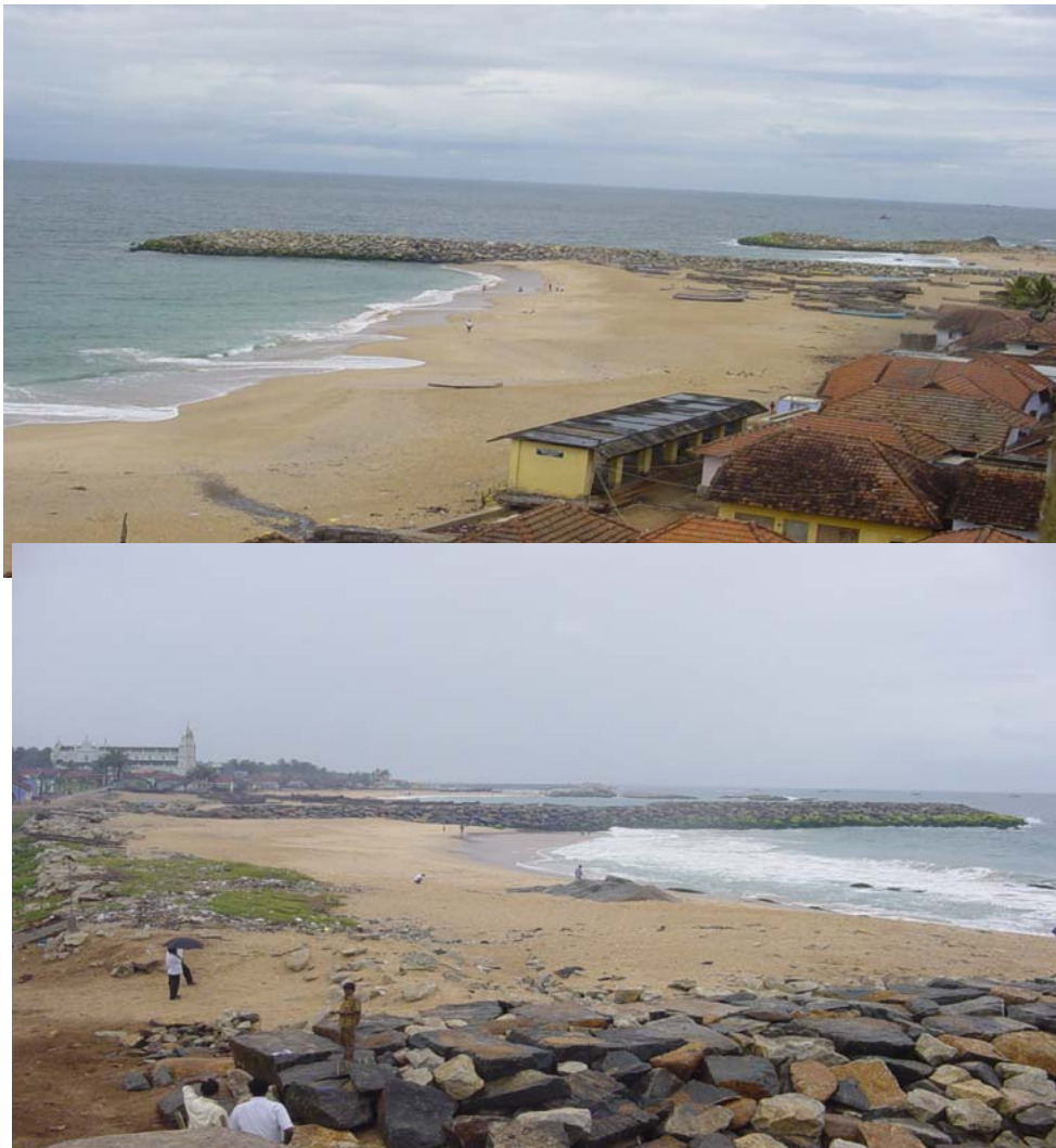
Photo.1.11. Effect of groins as an effective coastal protection measure (Kankumari District)
