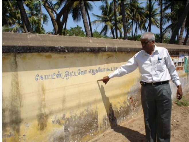
Photo 4.4 Watermark on a compound wall 1 Km away from Shoreline at Nagoor
