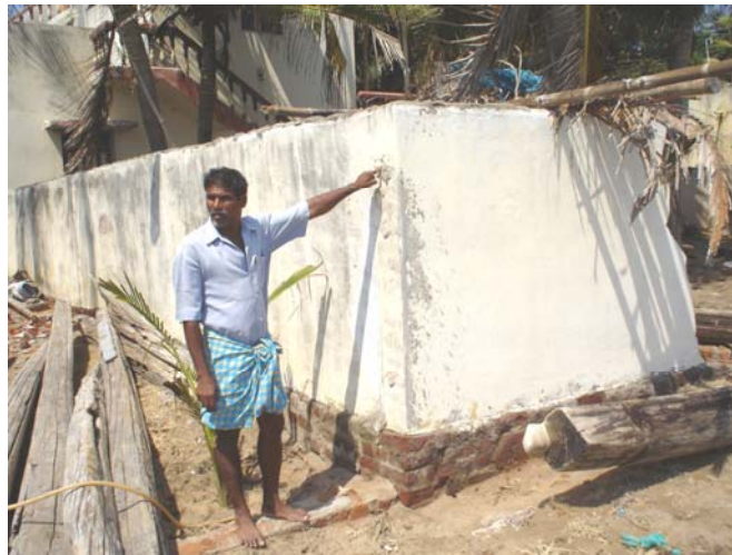
Photo 2.14. A local villager showing the tsunami run-up mark on the compound wall
