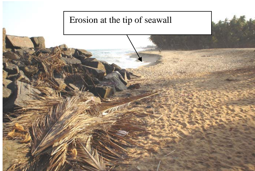
Photo 2.27. Erosion near the seawall at Nadukuppam
