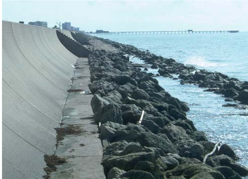
Photo. 1.1 View of a typical concrete seawall
