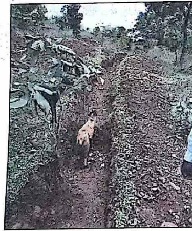
The trenches are 10 metres long, 3 metres deep, and just over a half metre wide; Each house in the village has a soak pit that facilitates water absorption.
