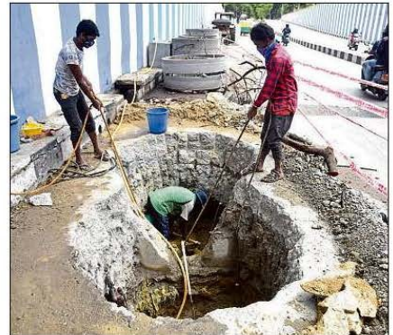
Storm water collection well being dug at Tagore Circle.
