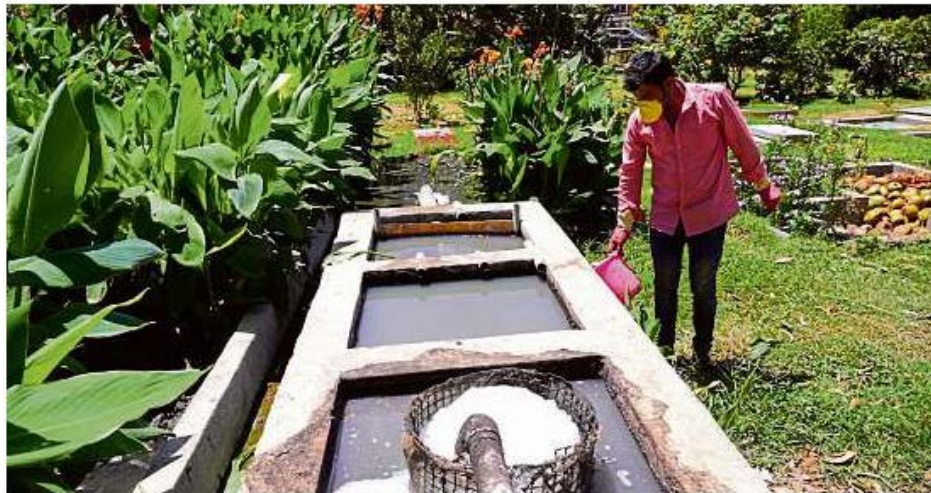
A phytotrid sewage treatment plant setup at Rainbow Drive Layout, Bengaluru. DH PHOTOS
