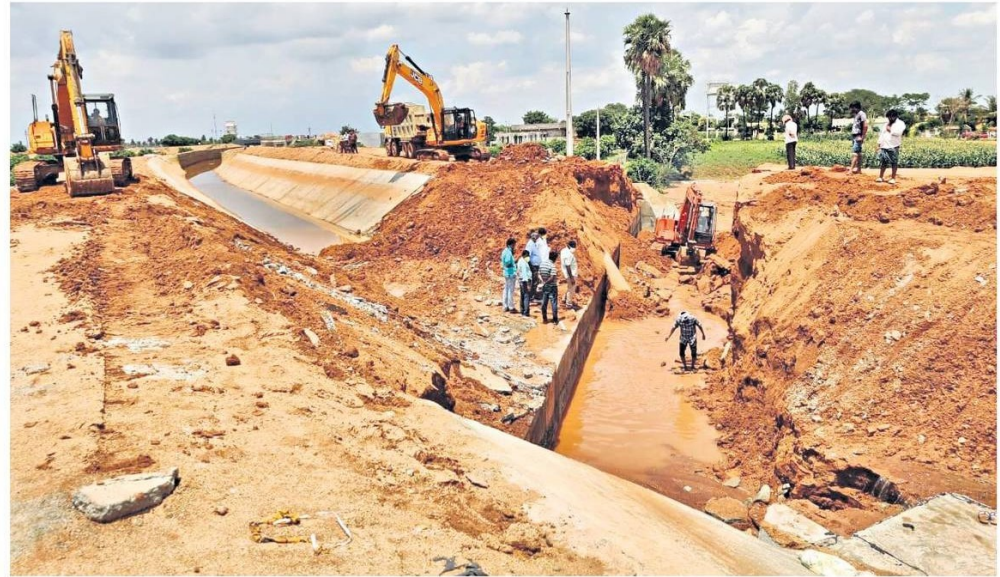
Filling work being taken up to plug the breach to the Jagadevpur canal of Kondapochamma Sagar, in Markook mandal of Siddipet.
