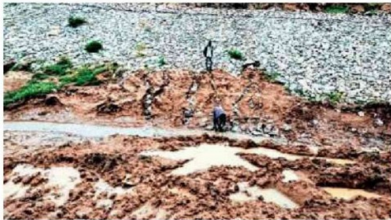
New worry: Water leaking from the Kondapochamma reservoir at Markook, Siddipet district, on Monday. ■ MOHD ARIF
