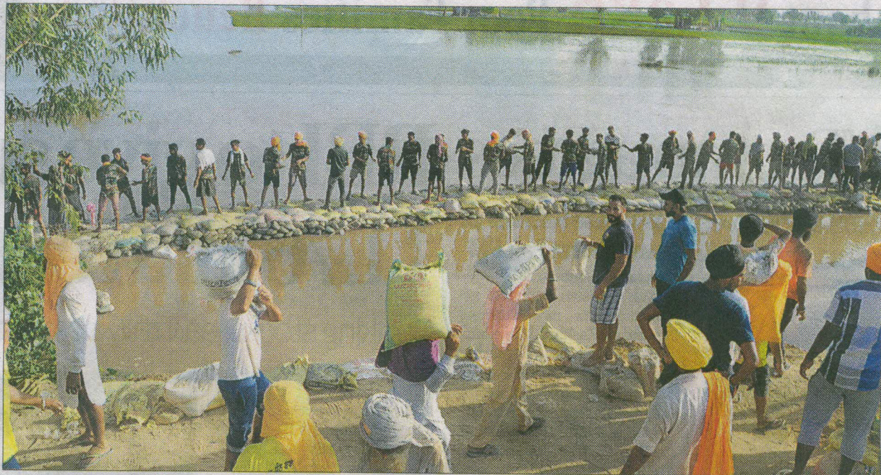
Volunteers carry sandbags and stones to plug the breach at Janian Chahal village in Jalandhar on Monday. PHOTO: SARABJIT SINGH
