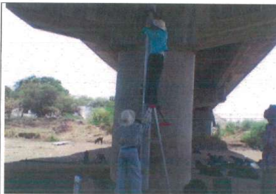
Fig.20: The Pressure Sensor is Anchored Firmly to the Pillar of the Bridge
