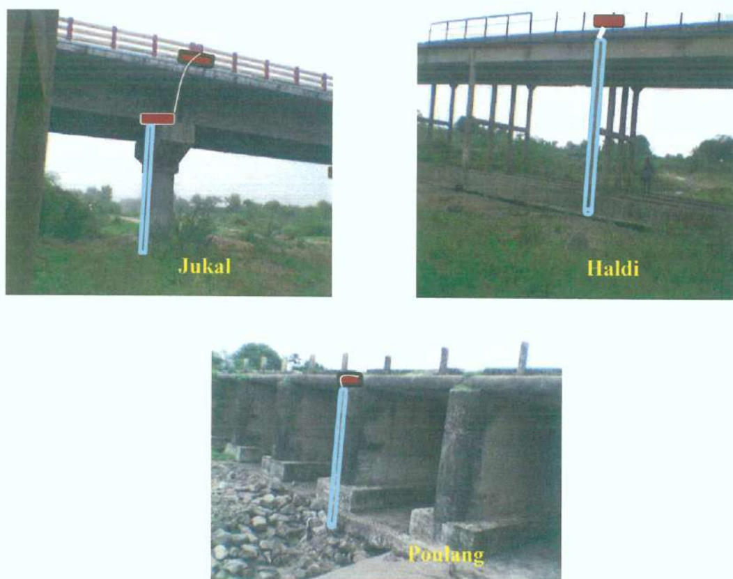
Fig.18: Installation of Automatic Water Level Recorder on Streams
