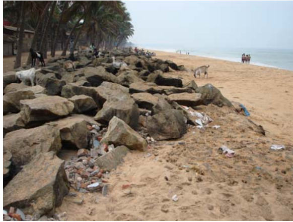
Photo 2.7. Damages to seawall at Beemapally
