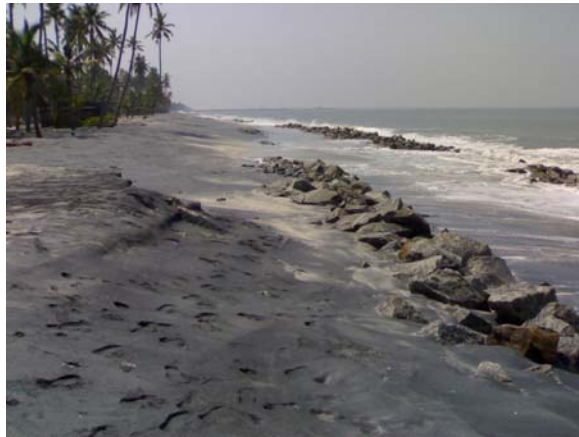
Photo.3.26 Remains of the seawall near Kayamkulam
