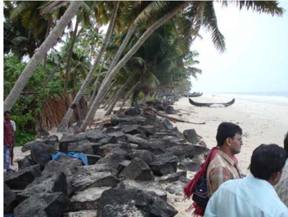
Photo. 4.19. Breached seawall at Andhakkaranazhy south
