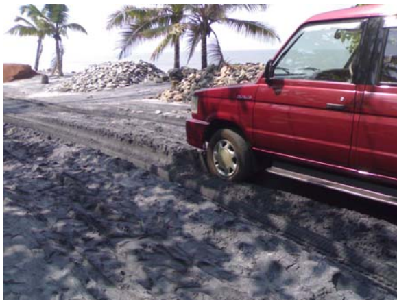
Photo.3.27 Overtopping of sand over the existing seawall near Kayamkulam
