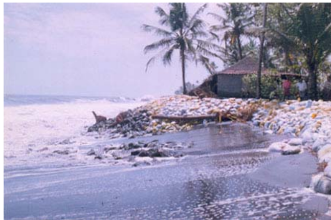
Photo.3.29 damage to existing seawall near Kayamkulam during storm
