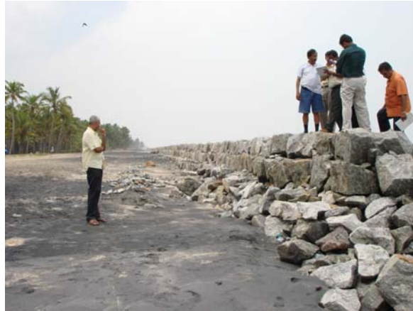
Photo 3.19. Damages to the seawall due to overtopping at Srayikadu
