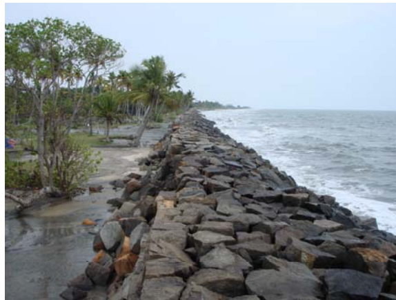
Photo 5.13. shows continious seeping of sea water through Seawall
