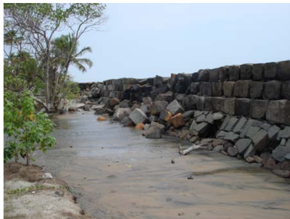
Photo 5.12. shows continuous seeping of sea water through Seawall
