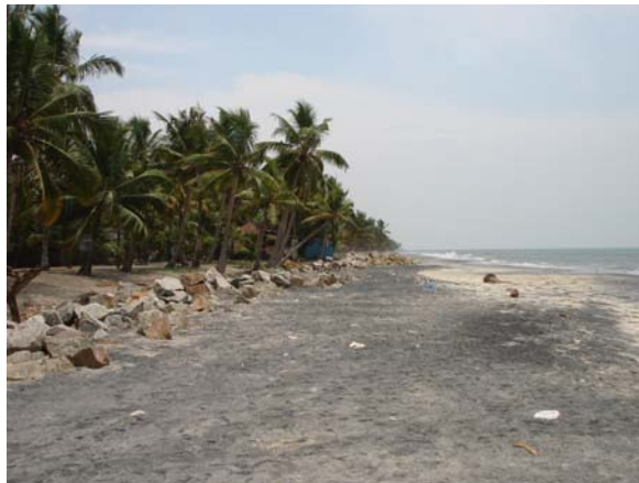
Photo 3.27. Extent of damage caused to the seawall South of Pathiankara
