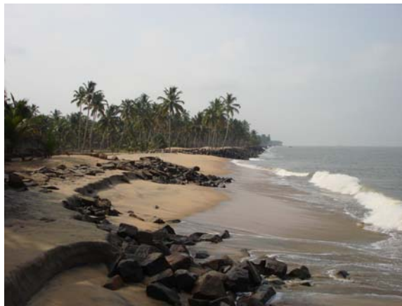
Photo 6.10. View towards south of Perinjinam showing the breached seawall
