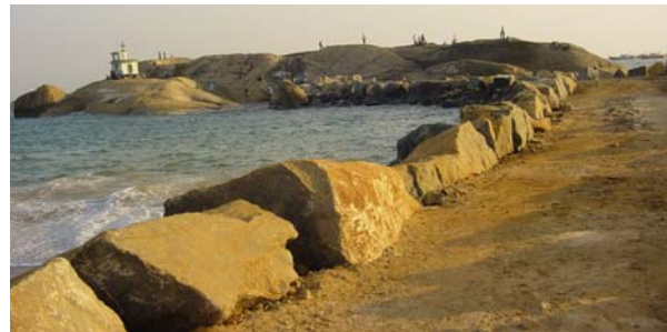
Photo. 5. A groin at Simon Colony (designed so as the natural outcrop acts as a head)
