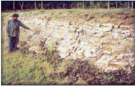
Checks with soil filled bags
