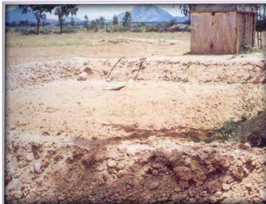
Lining of pond with white soil
