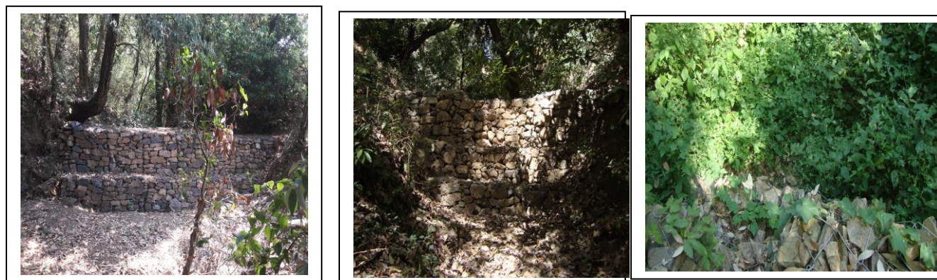
Plate 6: Gabion structure No. 1 and 2 and its impact in project area
