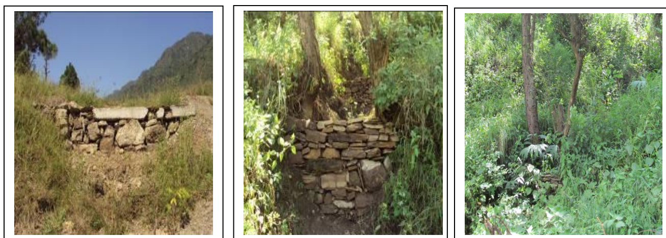
Plate 5: Loose boulder check dam and its impact in project area
