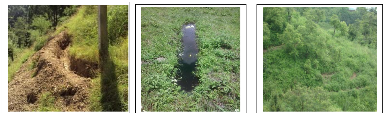
Plate 3: Trenches (Staggered) made and its impact in the project area
