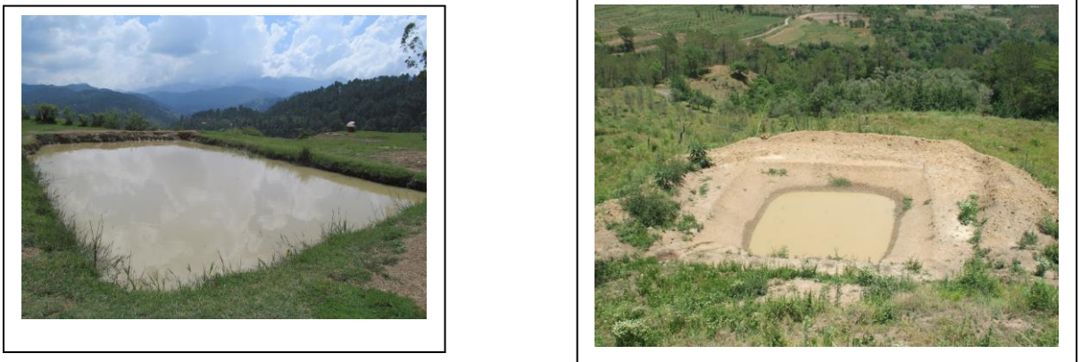
Plate 8: Renovation of earthen dam & Construction of LDPE farm pond – 50, 000 litres
