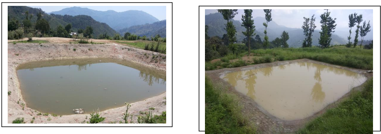
Plate 9: Construction of LDPE farm ponds (1,20,000 & 1,50,000 litres capacity)
