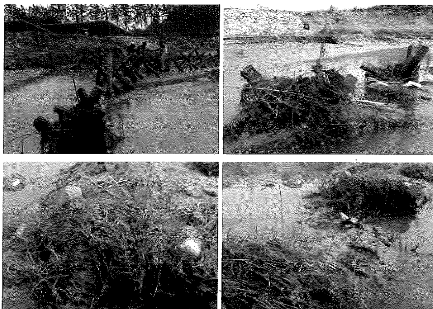
Figure 8.3 : Capturing of small trees and bushes in the jetty field in Solani River
