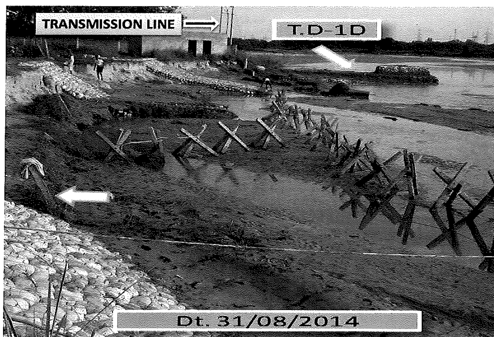
Figure 8.4 : Implementation of RCC Jack Jetty to inhibit further erosion between T.D-1 & T.D-1D
