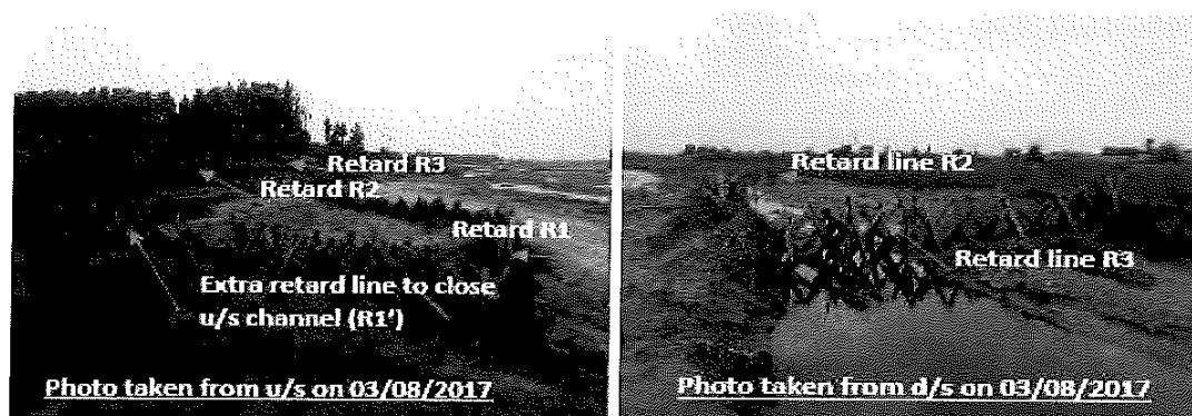
Figure 10.11 : Construction of Retard lines after channel formation
