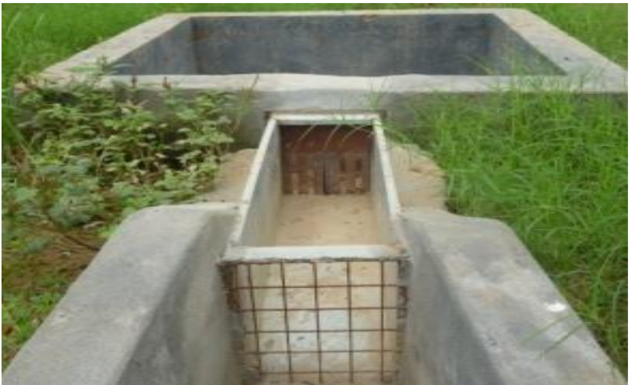
Figure 2.5 Conveyance Channel with Screen and Multi-Slot Divisor
