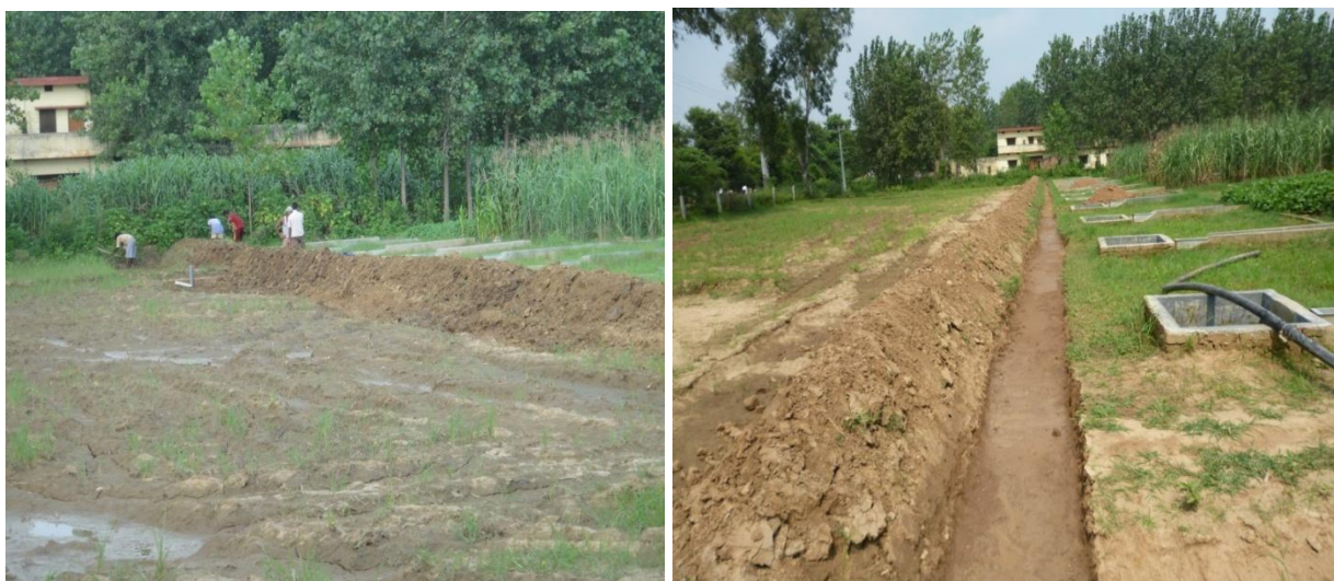
Figure 2.13 Construction of bund at farm for preventing the flooding at plots
