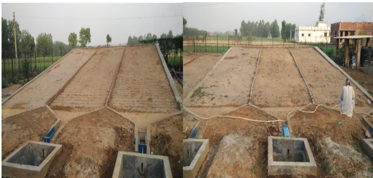
Figure 2.22 Construction of runoff collection tanks at the outlet of each plot
