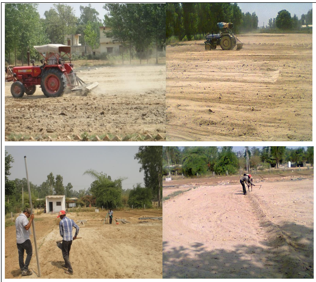
Figure 2.8 Slope fixing and demarking of plot after mixing of sandy soil
