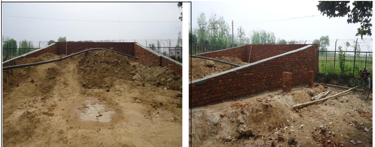
Figure 2.21 Snapshots of Masonary work for plot having Slopes 16%.
