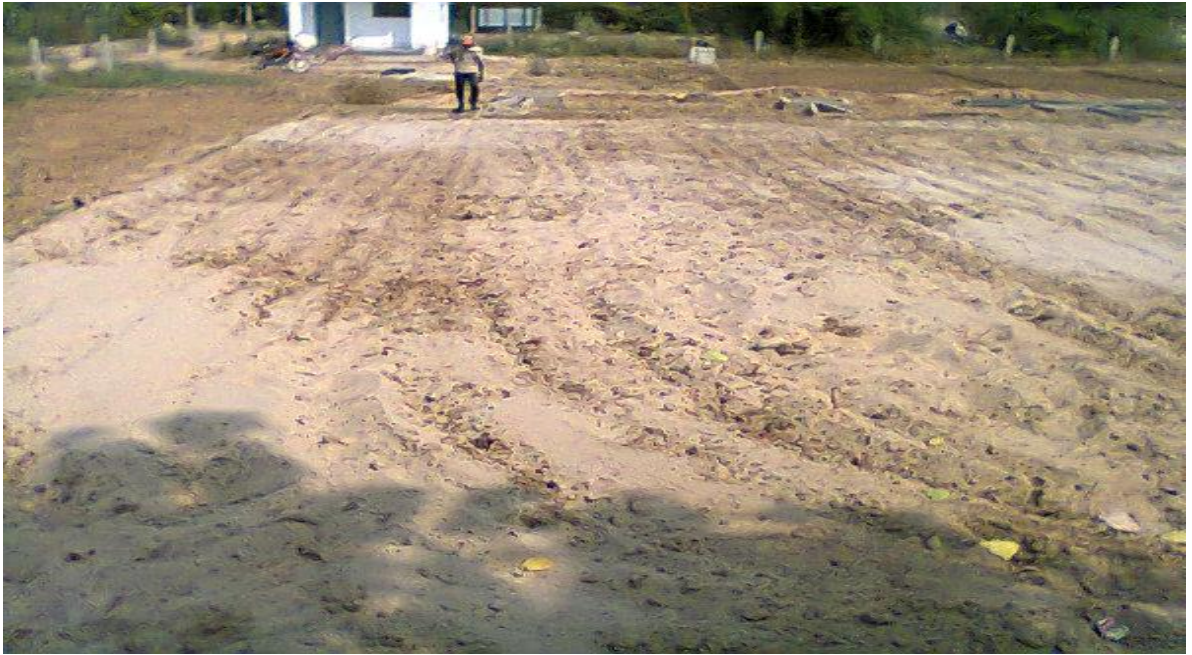
Figure 2.6 Addition and mixing of Sandy Soil to the Existing Soil
