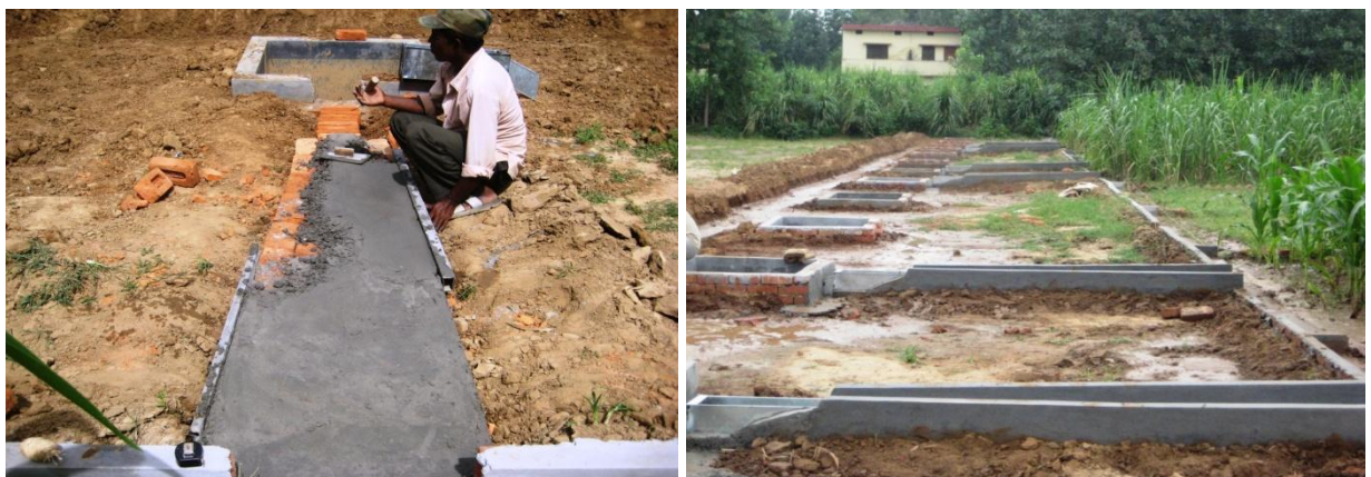
Figure 2.17 Construction of Approach Channel
