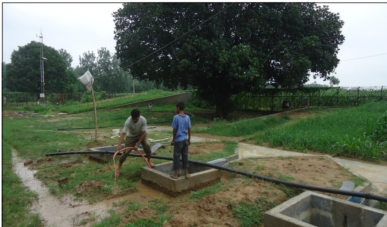
Figure 2.25 Construction of unlined small drain for preventing the flooding at plots.
