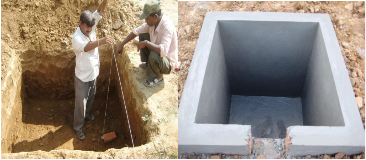
Figure 2.4 Runoff collection chamber constructed at outlet of maize plot
