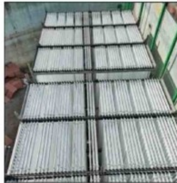
IFAS films being used to treat STP water with bacteria
