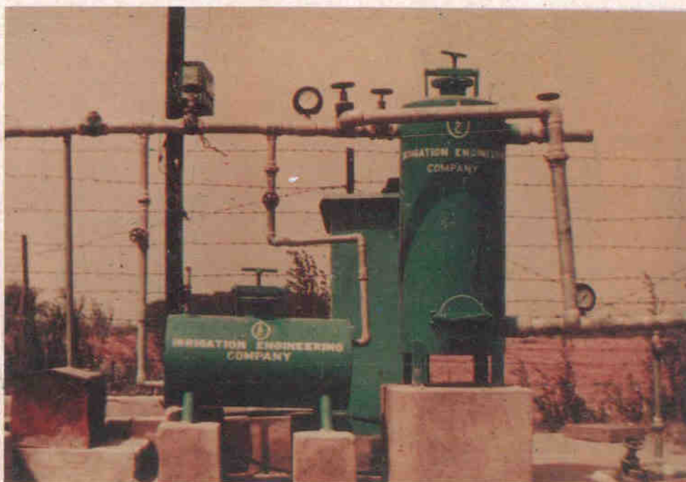
DRIP CONTROL ASSEMBLY WITH FERTILIZER TANK, SAND & SCREEN FILTER (Courtesy : WTC, IARI, New Delhi)
