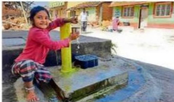
A recent survey of the functionality of tap connections under Jal Jeevan mission shows that 42% of the rural households in the state do not have fully functional tap water connections. DHNS/DTP
