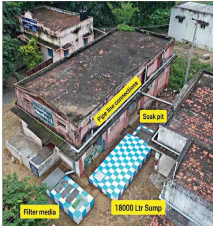
The harvesting structure allows the use of rainwater before it is let off into the soak pit
