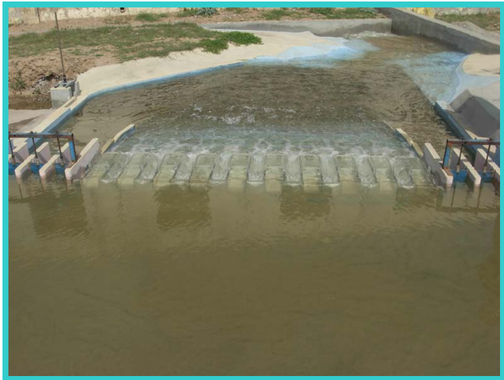
Plate No. 5.9 Running view of Piano Key Weir from u/s with under sluice gate
