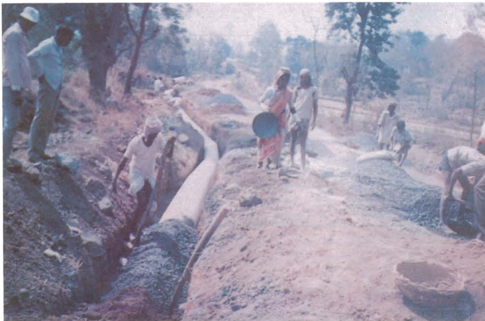
Concrete casing due to low depth at ch. 520 m.
