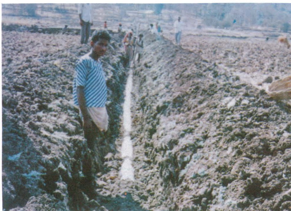
Filling trench lateral - 3, ch. 630 m.
