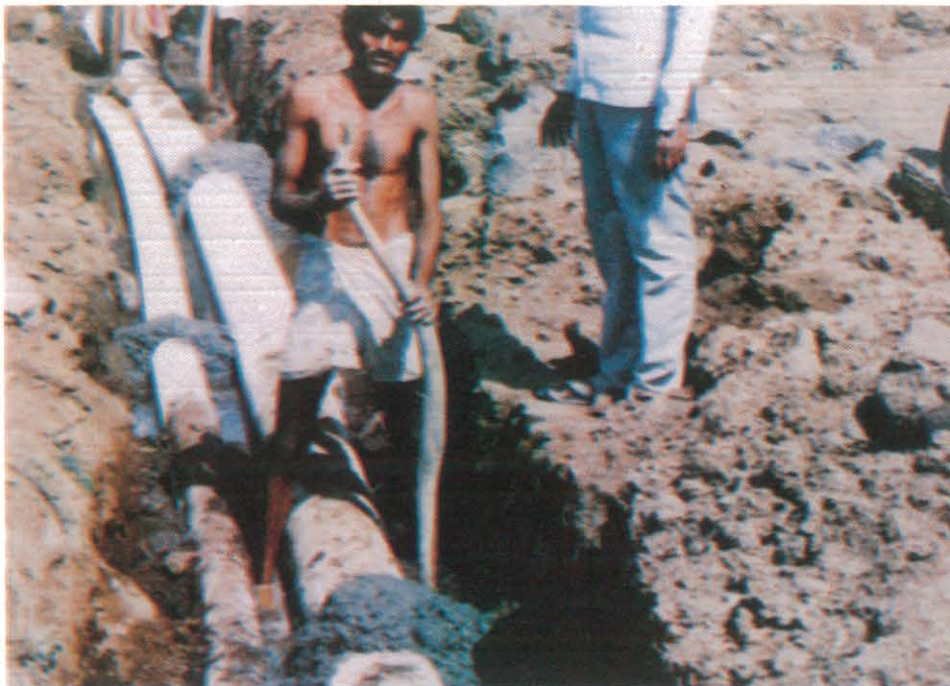
Hand compaction for lateral - I two parallel pipe line
