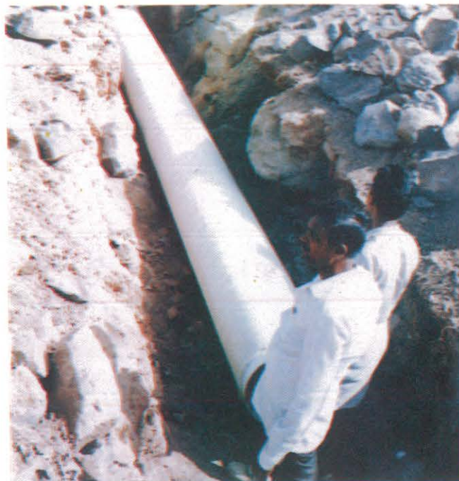
Jointing of Riblock Main Pipe Line at ch. 55m
