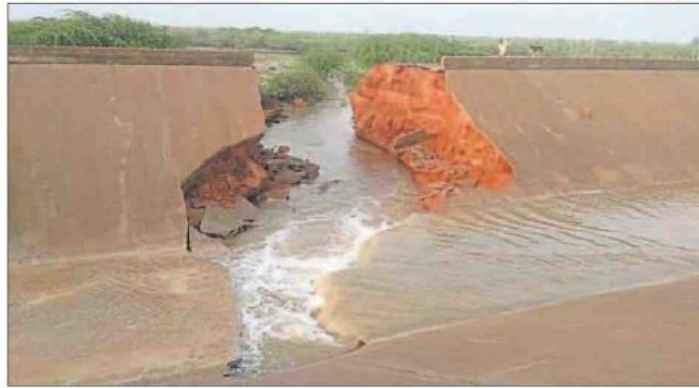
A breach in a patch of the Kutch Branch Canal project. HT PHOTO
