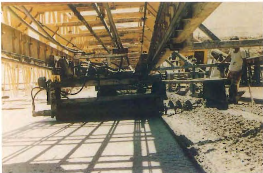
Photo - 2. C. C. Lining on Side Slope of Narmada Main Canal (NMC)
