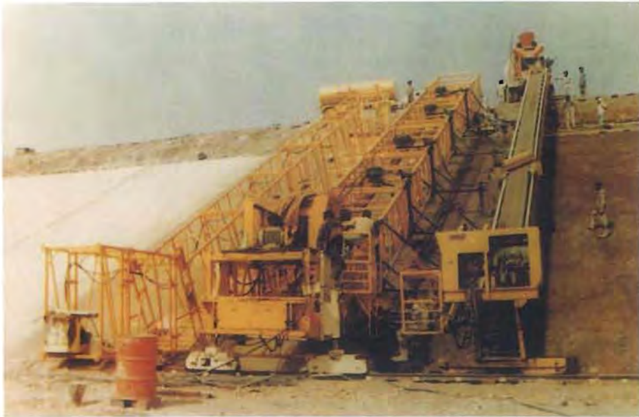
Photo - 1. C. C. Lining on Side Slope with Paver Machine (NMC)
