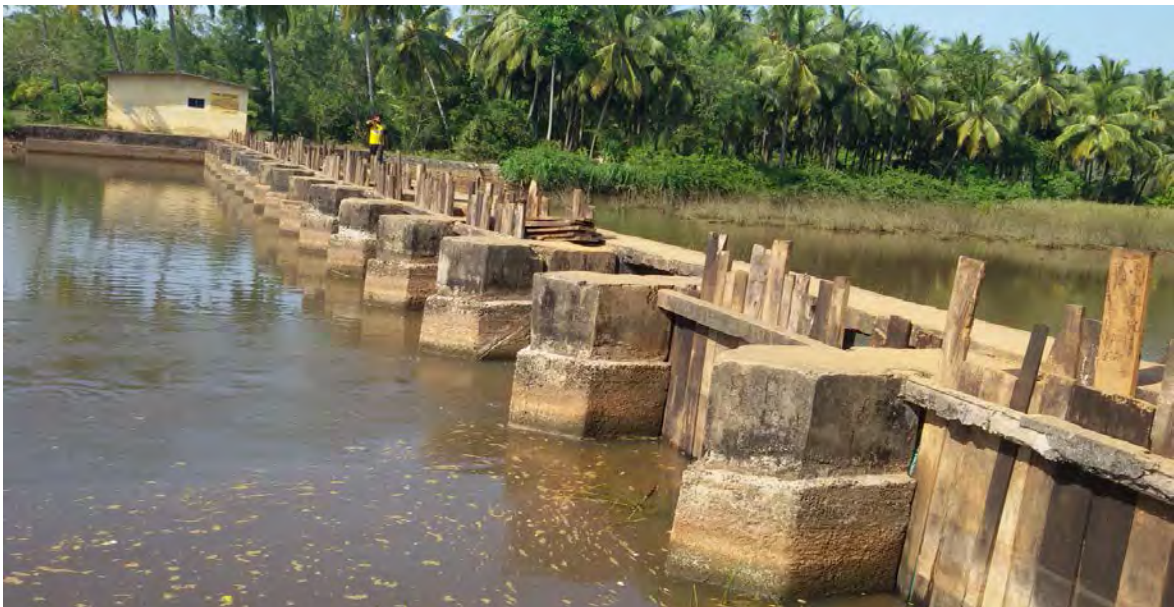
Figure 3.4.7 Salt water extrusion dam across Mogral River at Kottakkunje in Mogral Puthur Panchayat
