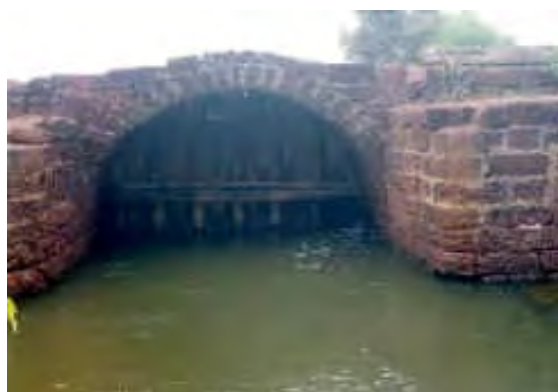
Closed sluice gate with wooden doors
