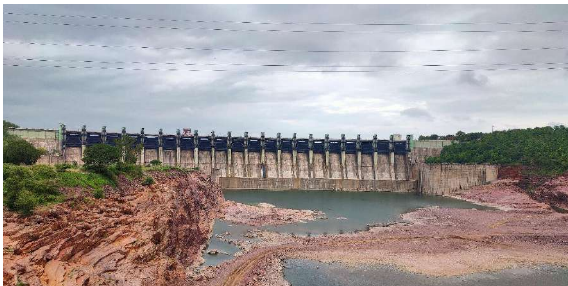
Photo 2: Indira Sagar Dam Spillway
