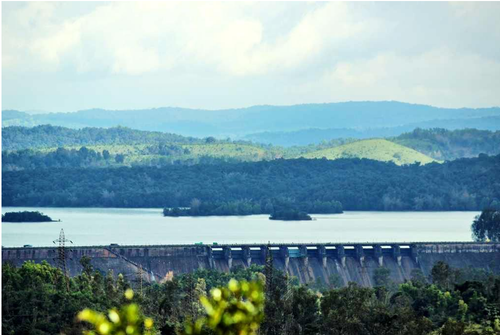
Photo 1: Tattihalla Dam reservoir
