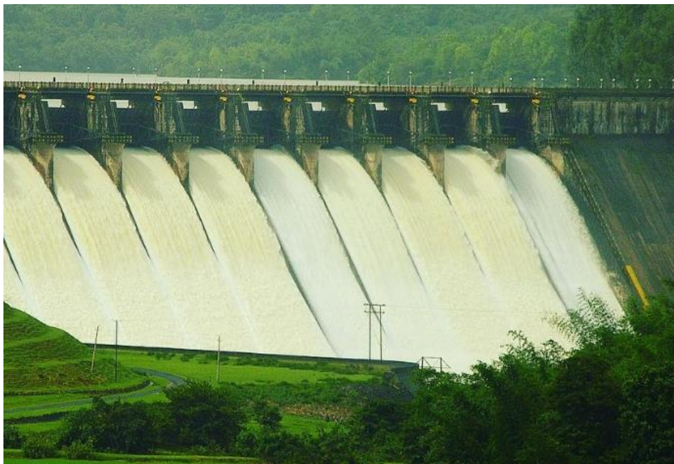
Photo 2: Tattihalla Dam Spillway
