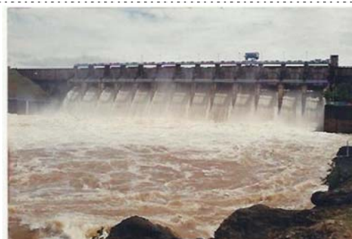
Figure 1. Tawa Dam in M.P., completed in 1974, is a 57.91-metre high composite dam that supplies irrigation water to a 246972-hectare command area.
