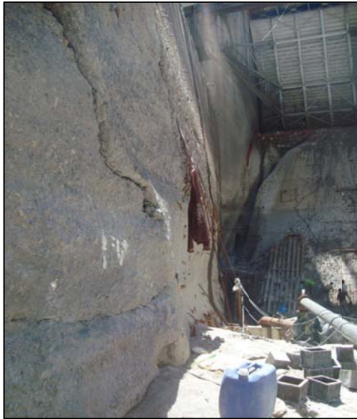
Figure 18. Energy dissipation erosion in overflow spillway at Maneri Dam in Uttarakhand. The spillway was eroded approximately five meters and set the stage for heavy remedial works.
