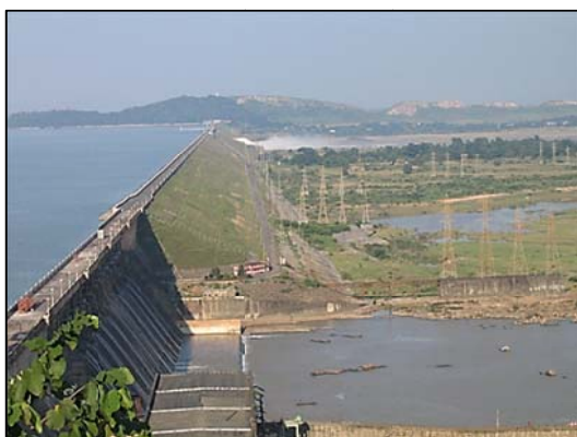
Figure 23. The revised inflow design flood for Hirakud Dam in Odisha requires and increased spillway capacity of 20,000 cubic metres per second.
