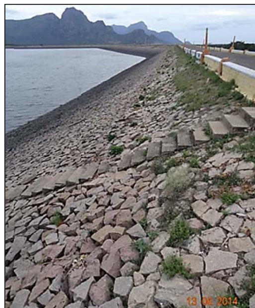
Figure 16. Displaced riprap caused by wave action on the upper slope of Thirumurthy Dam in Tamil Nadu.
