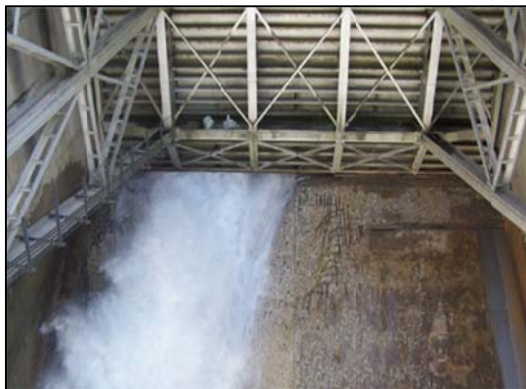
Figure 19. Spillway glacis beneath a radial gate at Ichari Dam in Uttarakhand has been eroded by abrasion from sediment resulting in significant leakage when the gate is fully closed.
