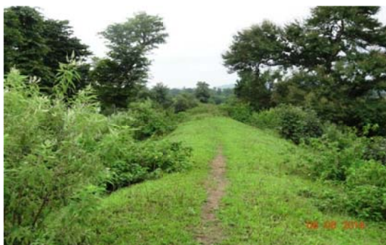
Figure 17. Woody vegetation inhibits dam safety inspection of Dhuty Weir located in Madhya Pradesh. Uprooted trees on the waterside of the dyke have over steepened the waterside slope resulting in large voids and reduced freeboard; and have reduced necessary x-section of the dyke for maintaining stability.
