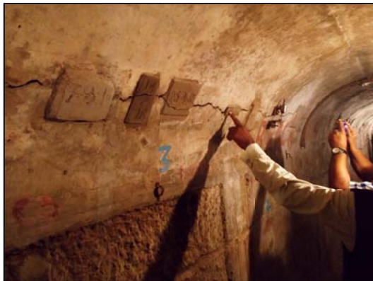
Figure 8. Cracking caused by repeated thermal stresses in the gallery of Konar Dam, a composite concrete-gravity/earthen-embankment dam located in Jharkhand.
