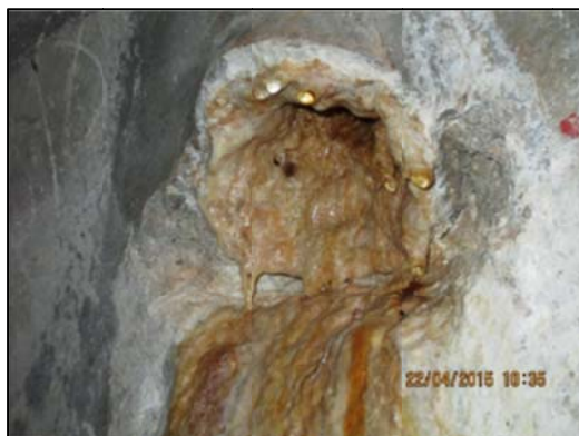
Figure 4. A clogged drain pipe at Ponnudi Dam in Kerala caused by increasing leakage and lack of maintenance. The reduction in flow through a pipe because of clogging can promote piping and lead to eventual collapse of a dam.
