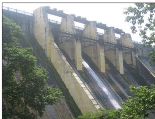
Figure 26. Chimoni Dam in Kerala has been thoroughly investigated for dam body seepage through 3D Sonic Tomography and is being rehabilitated by large scale grouting.
