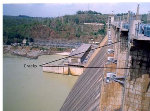
Figure 5. Large cracks have developed in Rihand Dam in Uttar Pradesh as the result of alkali-aggregate reaction.
