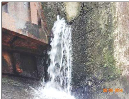
Figure 10. Leakage downstream of vertical lift gate coming from a deteriorated horizontal lift joint at Ichari Dam in Uttarakhand.
