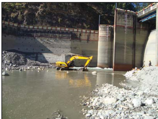
Figure 20. Excessive sediment accumulation in reservoirs, particularly near the intakes of bottom outlets, such as at Maneri Dam in Uttarakhand shown here, can be mobilized quickly when gates are opened and obstruct flow through the outlet.
