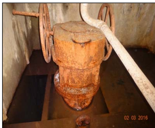
Figure 21. A sluice gate valve at Barna Dam in Madhya Pradesh that has not been operated in many years. Sediment deposits in the reservoir have blocked the sluice inlet.
