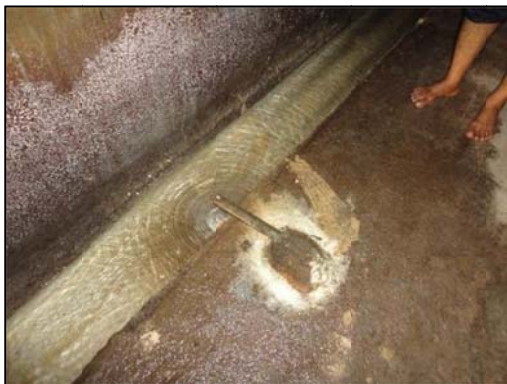
Figure 6. A flooded gallery and leachate stains at Karanja Dam in Karnataka. The presence of leachate indicates chemical reactions between reservoir water and dam body materials.
