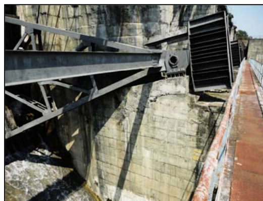
Figure 22. Leakage and flaking of concrete beneath the trunion of a radial gate at Bennithora Dam in Karnataka because of deterioration of lift joints from large daily temperature variations and chemical action.
