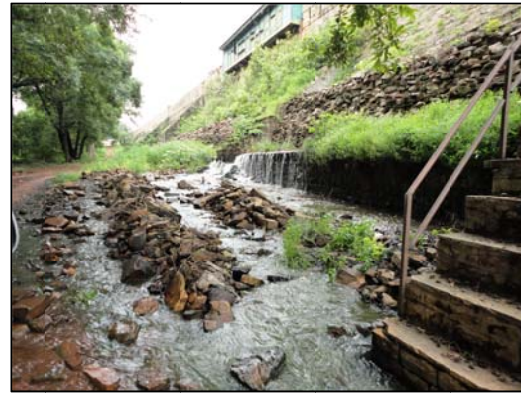
Figure 7. Masonry gravity dams are subject to leakage caused by failed mortar and construction joints, and by the growth of plant roots that create paths along which water can flow easily, such as at Chandpatha Dam in Madhya Pradesh. Large seepage flows can remove internal material, resulting in catastrophic failure.
