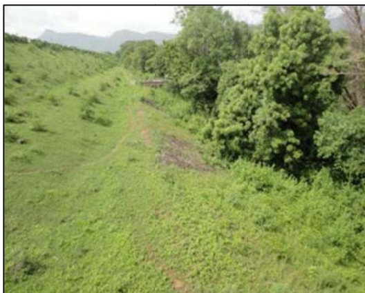
Figure 14 Large trees allowed to grow on the downstream embankment slope of Meenkara Dam in Kerala make visual detection of seepage difficult and can promote leakage along the paths of roots extending into the dam.
