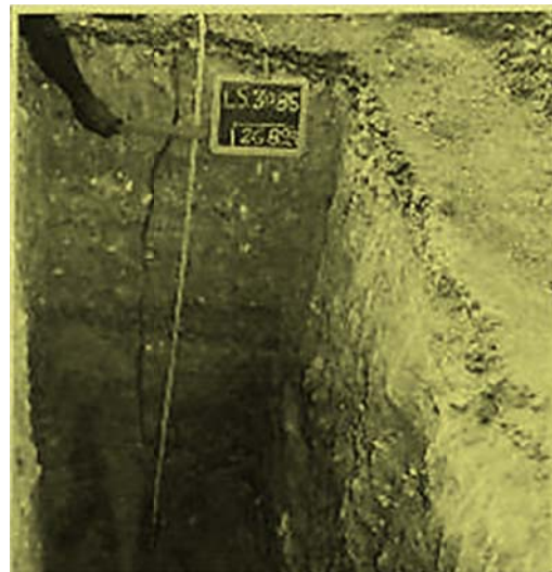
Figure 11. Differential settlement of impervious shoulder resulting in longitudinal crack forming at the dam top above the clay core as seen inside the trench; Upper Tiruppur Dam, Tamilnadu.
