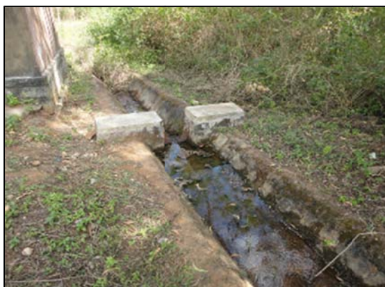
Figure 12. Leakage is monitored by collecting seepage water in discharge channels and measuring the flow using small weirs. At some DRIP dams measuring weirs have been damaged or removed making assessment of dam deterioration by internal erosion impossible. The measuring weir at Balimela Dam in Odisha shown in the photograph is open to the environment, unprotected, and vulnerable to damage.
