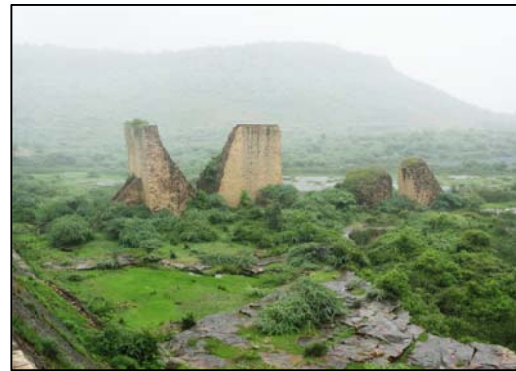
Figure 3. Tighra Dam in Madhya Pradesh is a masonry gravity structure built in 1916 for agricultural irrigation and municipal water supply. The dam failed on the afternoon of Aug 4, 1917 during a large flood because of a weak foundation that could not resist the hydraulic pressure. The dam was repaired and is in operation today.
