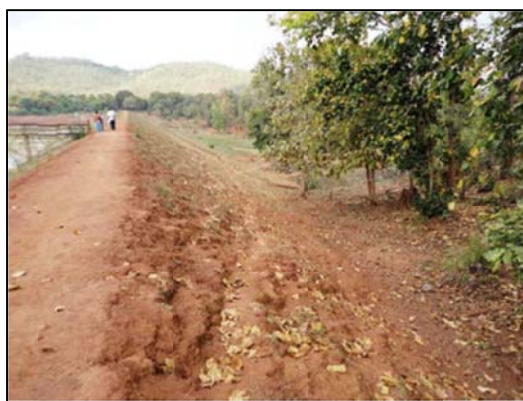
Figure 15. Surface erosion on downstream embankment of Balaskumpa Dam in Odisha. Note the absence of grass cover that would prevent soil erosion on the embankment slope.
