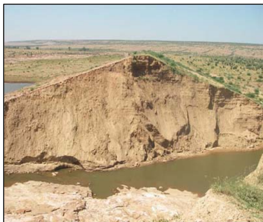
Figure 13. Gararda Dam in Rajasthan breached during the very first filling on Aug 15, 2010 because of internal erosion along the embankment/foundation interface.
