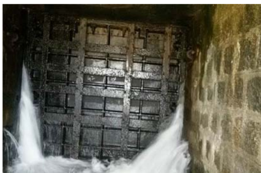
Figure 27. Profuse leakage from the aged gates of the Krishna Raja Sagar Dam, Karnataka
