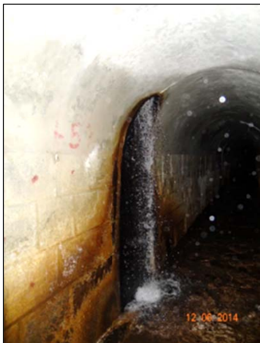
Figure 9. Leakage at contraction joints are typical in most masonry dams indicating failed or defective waterstops, such as shown here in the gallery of Upper Bhavani Dam in Tamil Nadu
