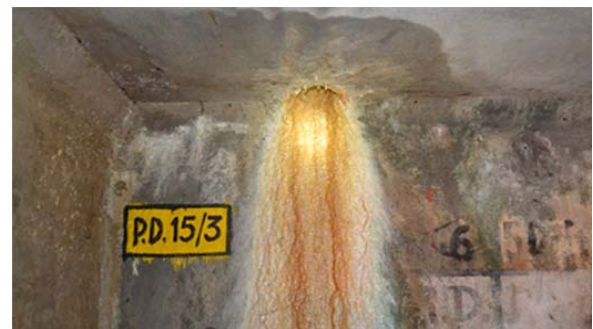
Figure 7 - Clogged drain at Barna Dam, MPWRD
