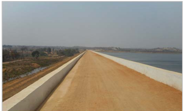
Rip-Rap, toe drain and parapet wall repairs at Kelavarapalli Dam, TNWRD
