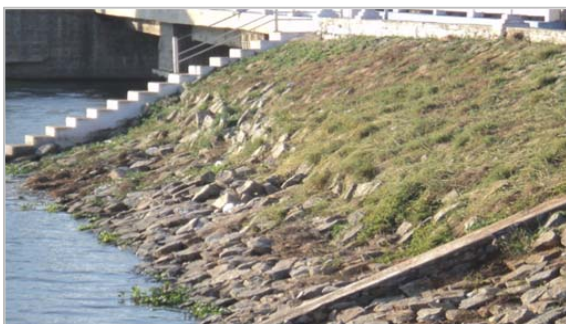
Rip-Rap, toe drain and parapet wall repairs at Kelavarapalli Dam, TNWRD
