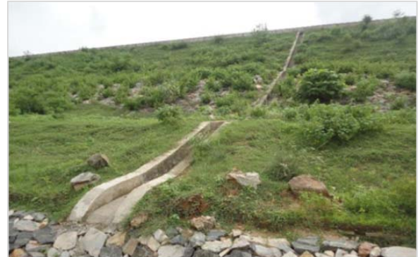
Figure 5 - Excessive vegetation at Derjang Dam, OWRD
