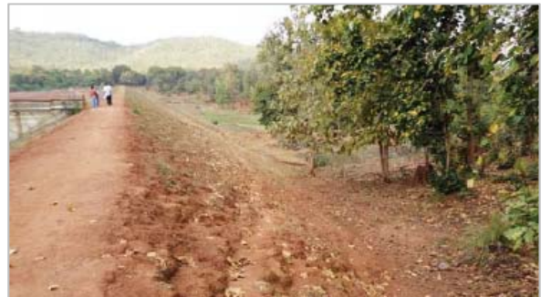
Figure 6 - Surface erosion of d/s face at Balaskumpa Dam, OWRD
