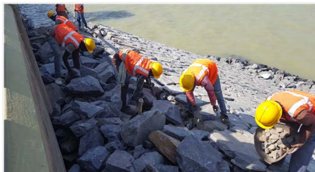
Figure 12 – Rip-rap work at Maithon Dam, DVC, Jharkhand
