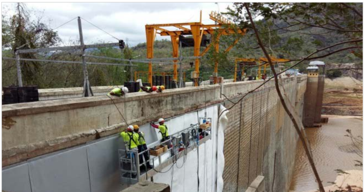
Figure 11 - Placing of geo-membrane, Servalar Dam, TANGEDCO
