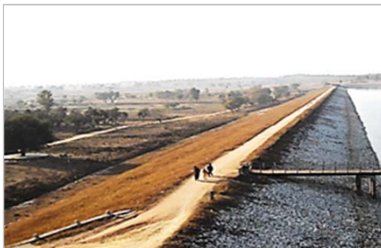
Rip-Rap, toe drain and parapet wall repairs at Kelavarapalli Dam, TNWRD
