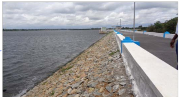
Rip-Rap, toe drain and parapet wall repairs at Kelavarapalli Dam, TNWRD
