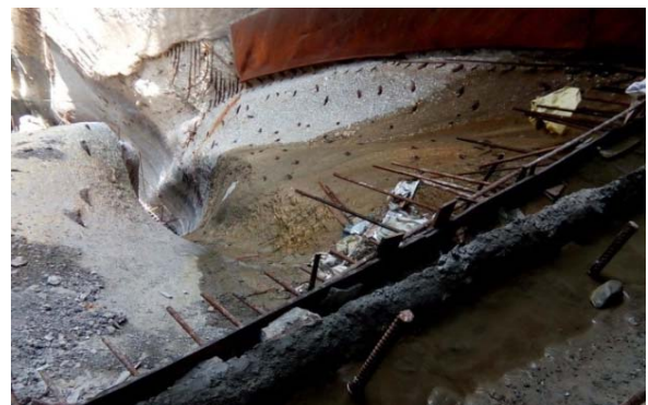
Figure 8 – Abrasion of spillway at Maneri dam, UJVNL
