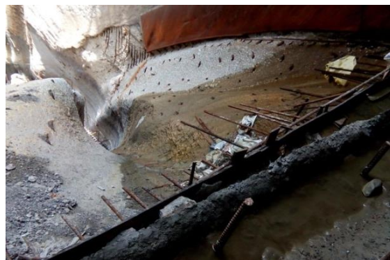
Figure 8 – Abrasion of spillway at Maneri dam, UJVNL
