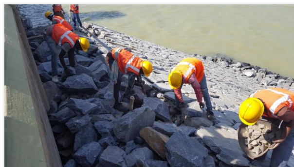
Figure 12 – Rip-rap work at Maithon Dam, DVC, Jharkhand
