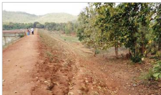
Figure 5 - Excessive vegetation at Derjang Dam, OWRD
