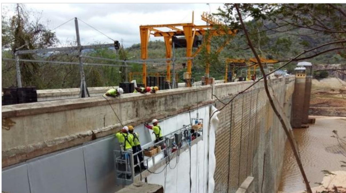
Figure 11 - Placing of geo-membrane, Servalar Dam, TANGEDCO
