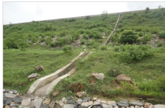
Figure 5 - Excessive vegetation at Derjang Dam, OWRD
