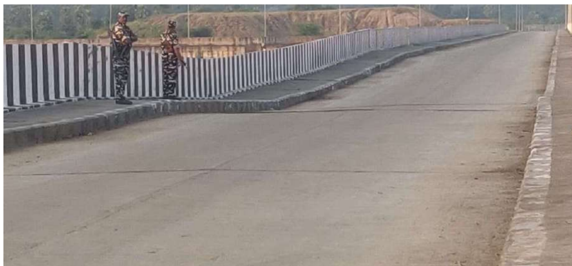
Deck Slab Deflection at Pier 20 of 7 th Block
