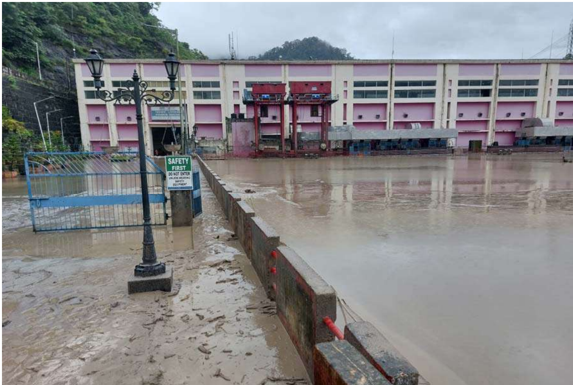
Fig.-6 TLDP-III D/s view of power House. Silt and slush deposit on TRC
