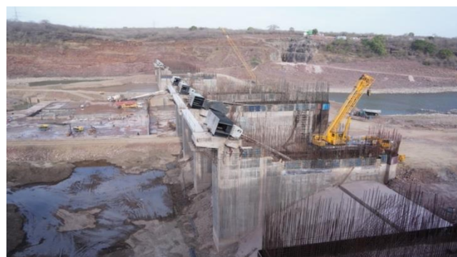
Fig. 5.6: Parwan Dam, Rajasthan
