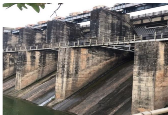
Fig. 5.13: Spillway of Soundur Dam
