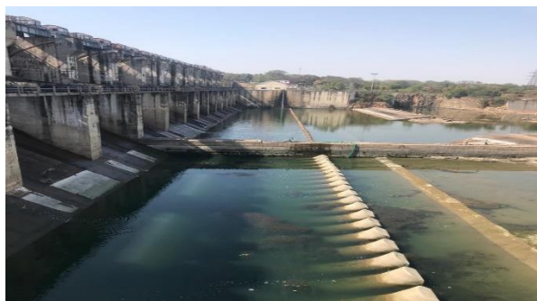
Fig. 5.12: Energy Dissipation Arrangement of Ravisankar Sagar Dam
