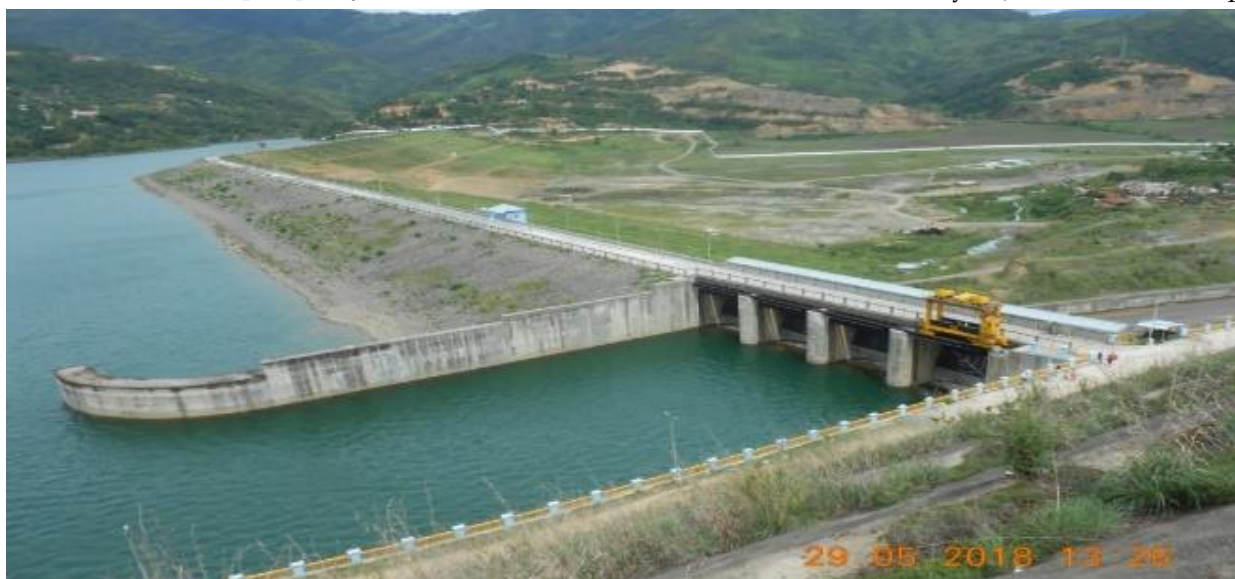
Fig. 2.4: Thoubal Multipurpose Project, Manipur (Project under PMKSY-AIBP)
