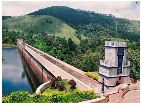
Fig. 5.14: Mulla Periyar Dam
