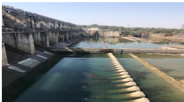
Fig. 5.12: Energy Dissipation Arrangement of Ravisankar Sagar Dam
