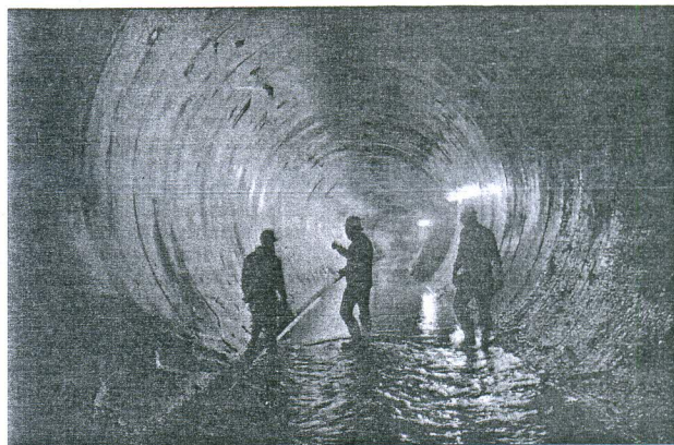
A section of the 23.24-km-long tunnel between Gurez and Bandipora, dug out by the Tunnel Boring Machine, providing all-weather access
