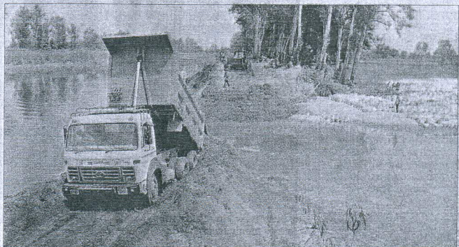
The breach in the Western Yamuna Canal being plugged on Tuesday. TRIBUNE PHOTO
