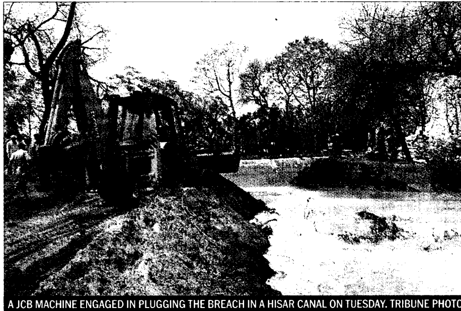
A JCB MACHINE ENGAGED IN PLUGGING THE BREACH IN A HISAR CANAL ON TUESDAY. TRIBUNE PHOTO
